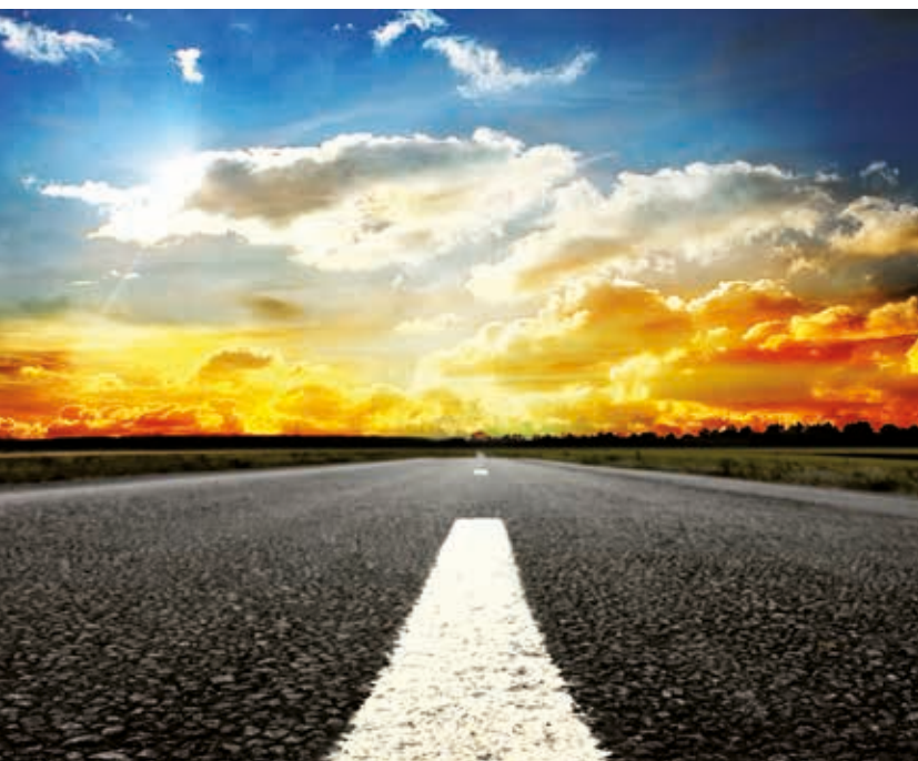
Brand new asphalt on a road
