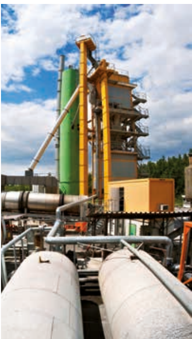
Asphalt production plant
