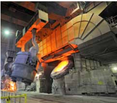
Steel production plant
