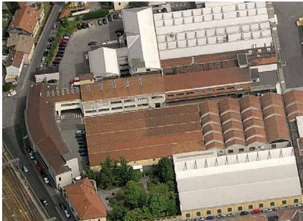
Testori Headquarters (Novate Milanese)
